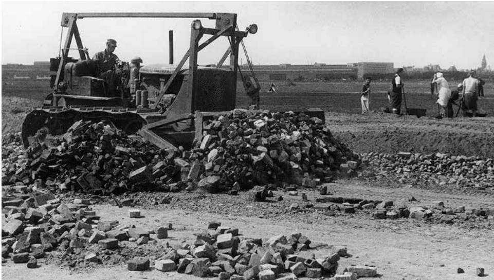
An Army engineer operates a bulldozer as German laborers clear the field with shovels to construct a new runway at Tempelhof.
